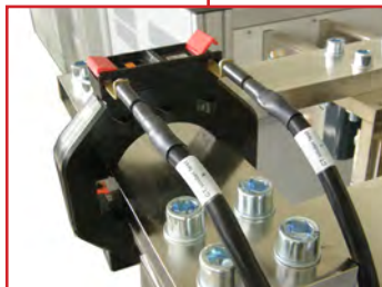
Detail of the CT under test connected at the secondary side.
